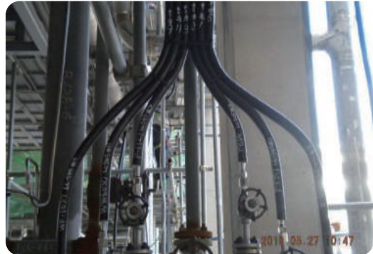
| STEAM TRACING CONSTRUCTION |
