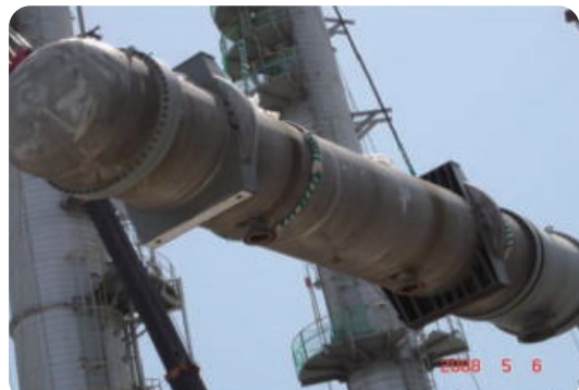
| REVAMPING PROJECT REACTOR INSTALLATION |
