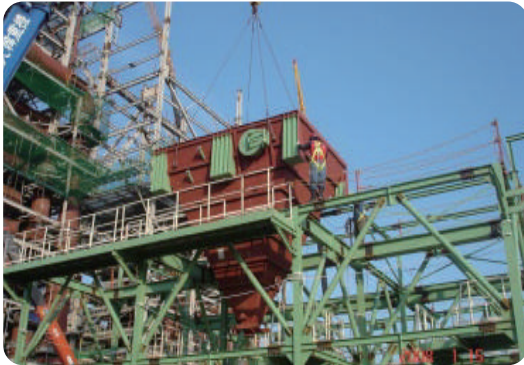
| CHP PROJECT DUST COLLECTOR INSTALLATION |
