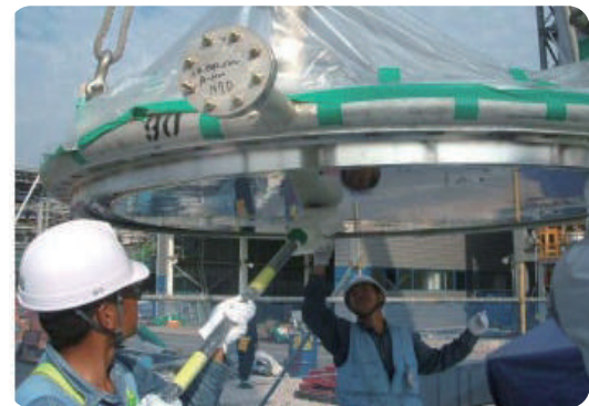
| INTERNAL HEADER INSTALLATION |
